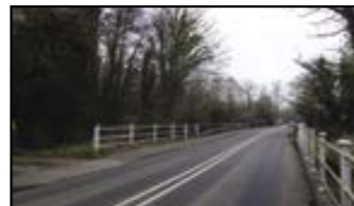
B3335 Highbridge Rd River Bridge
